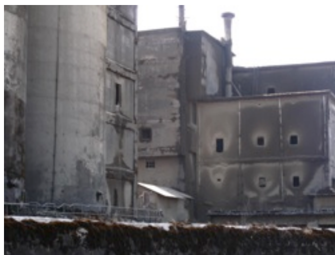
The cement works above Cherrapunjee Cave. Photo: Yoav Bar-Ness
